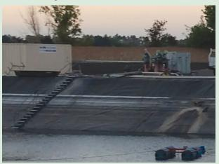
The Flexstep utilizes patented technology to produce a stairway with a unique combination of a pressure dissipating mat base, and adjustable steps that are also non penetrating to liners. The adjust-ability of stairway provides for safe and efficient access for many industrial applications.
